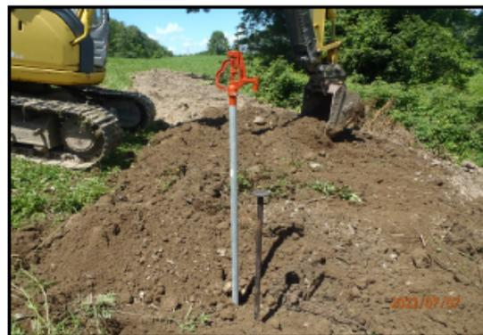
Figure 2. Completed frost-free hydrant with shut-off valve.
