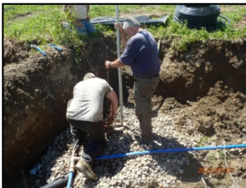
Figure 1. Contractor and farmer assembling the first frost-free hydrant.
