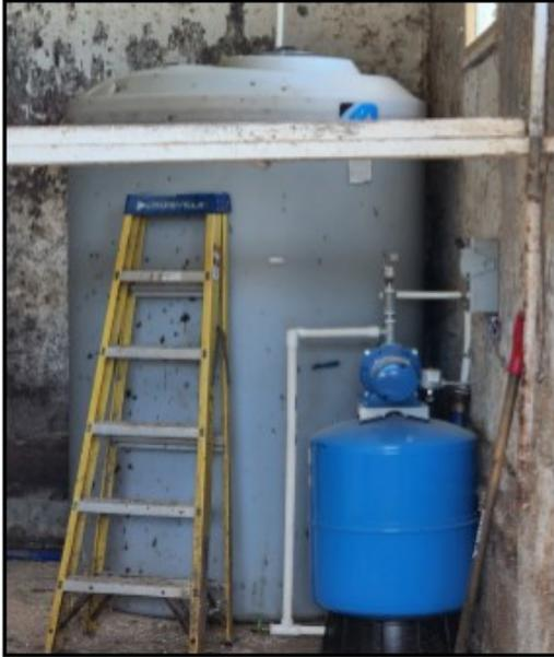
Figure 3. New holding and pressure tanks were installed because of conflicting pipe sizes between the barn and the watering system.
