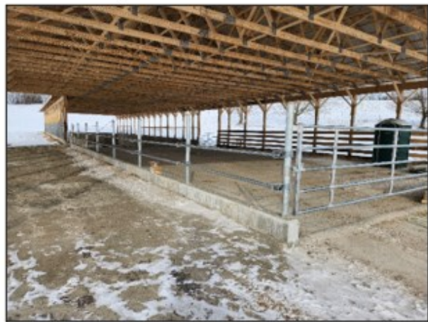
Figure 5. The covered barnyard with feed alley will allow the farm to capture the nutrients that were lost during rainstorms and a non-conductive cleaning surface.
