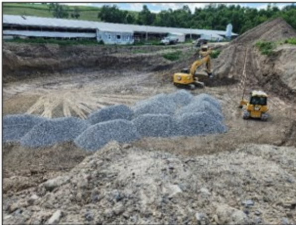
Figure 1. The contractor works on excavating the footer elevation.
