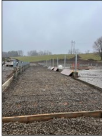
Figure 2. The contractor had prepared the feed alley for concrete.
