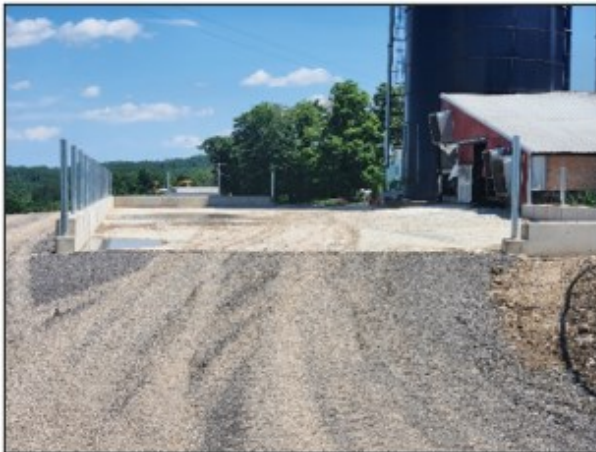
Figure 3. The newly constructed barnyard and push off area will be used to facilitate cleaning of the barn.
