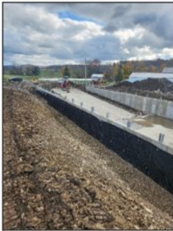
Figure 1. The monolithic footer and floor are poured for the manure storage.
